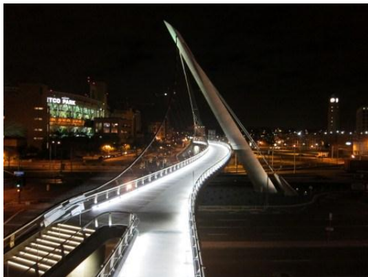
Harbour Drive Bridge, San Diego, USA
